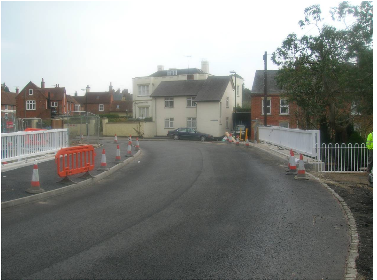
The New Bridge Looking East from Waterside Mill
