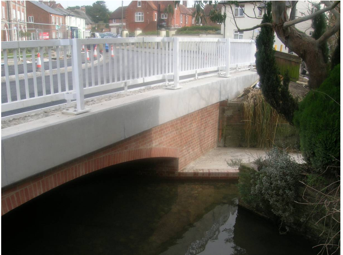
Span 1 – Southern Façade Adjacent to The Old Mill
