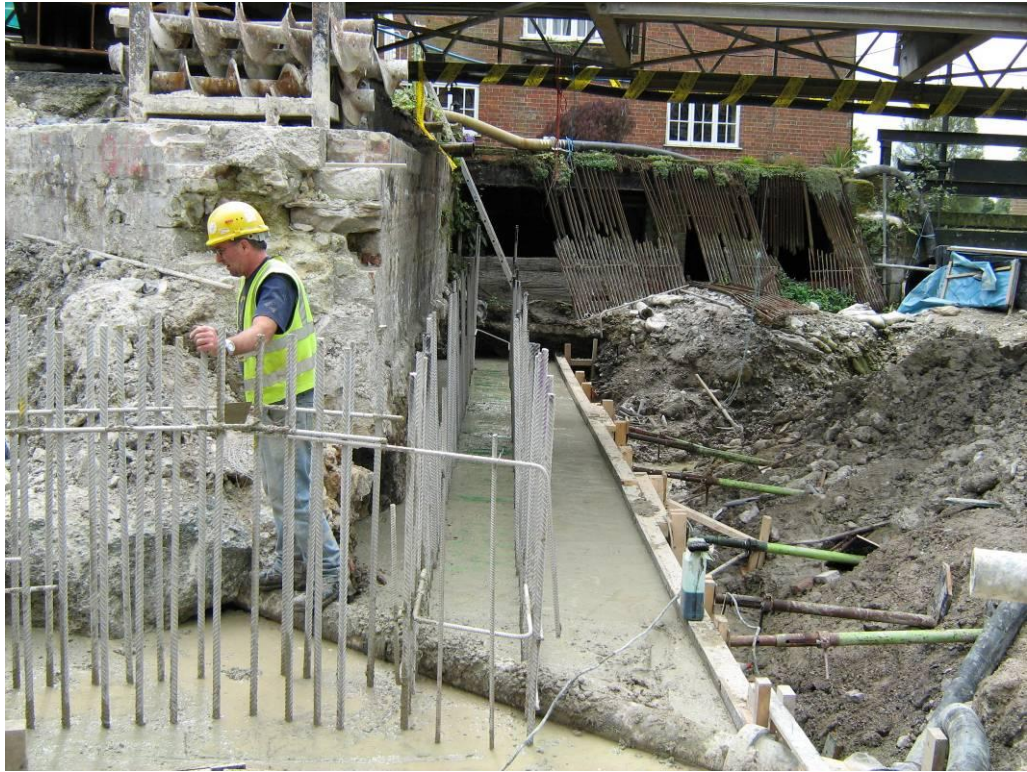
Photograph 2 Casting Operations to Central Triangle Showing Eastern Abutment – Span 2
