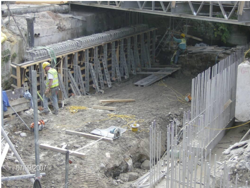
Photograph 1 Casting Operation to Span 1
