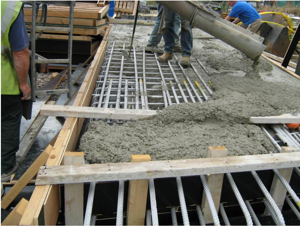
Photograph 4 'In Progress' Casting Operations to Precast Deck Units
