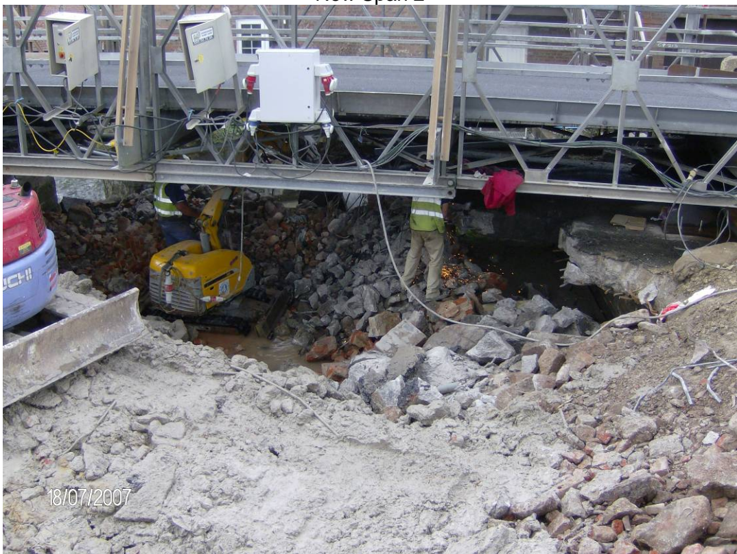
Photograph 2 Demolition Works to Spans 10/11
