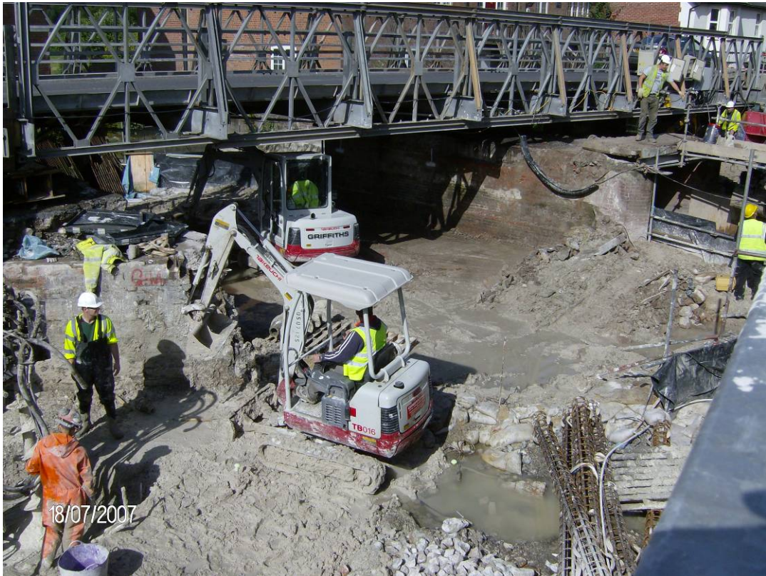
Photograph 1 General Site Operations New Span 2
