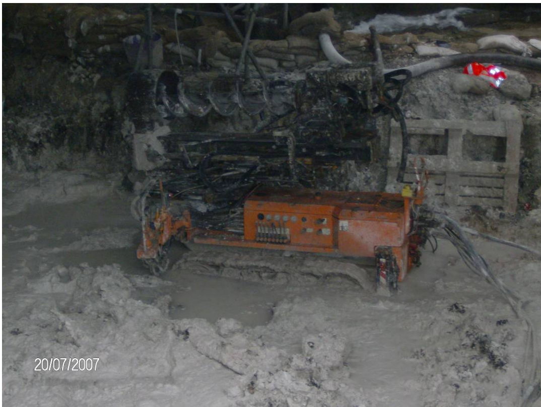
Photograph 4 Piling Operations in Span 1
