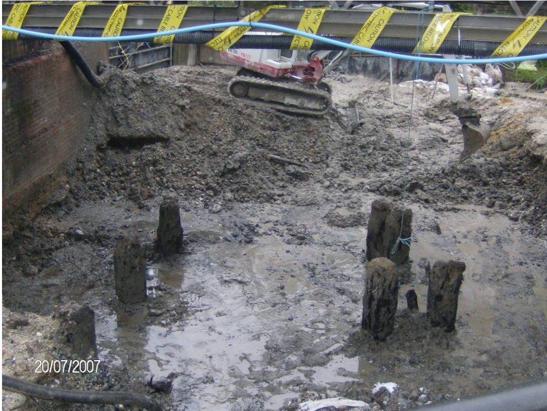
Photograph 3 Old Piles New Span 2 Taken from the Waterside Mill
