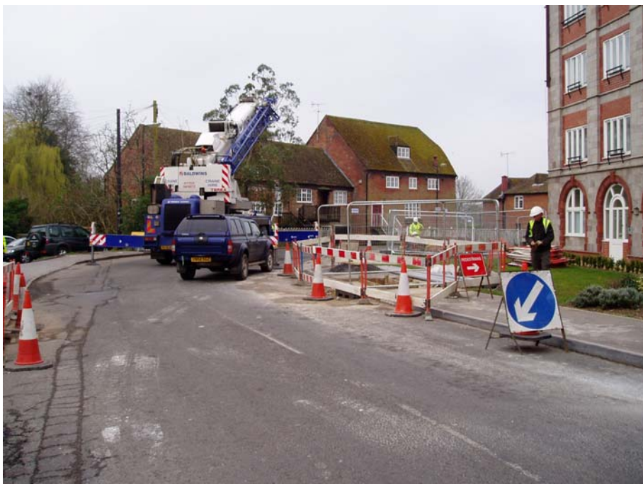
Photo 2 – BT trenches in The High Street
