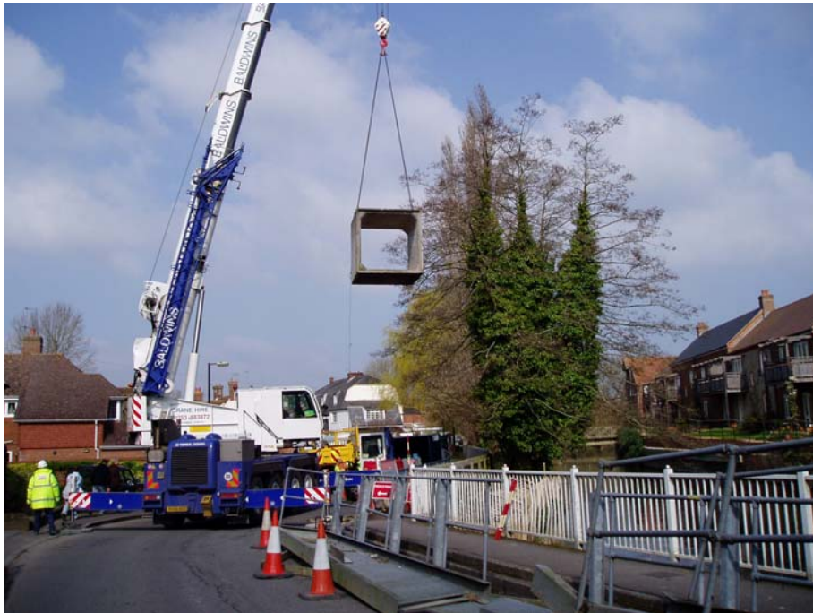
Photo 5 – Installation of footbridge centre pier (culvert units)
