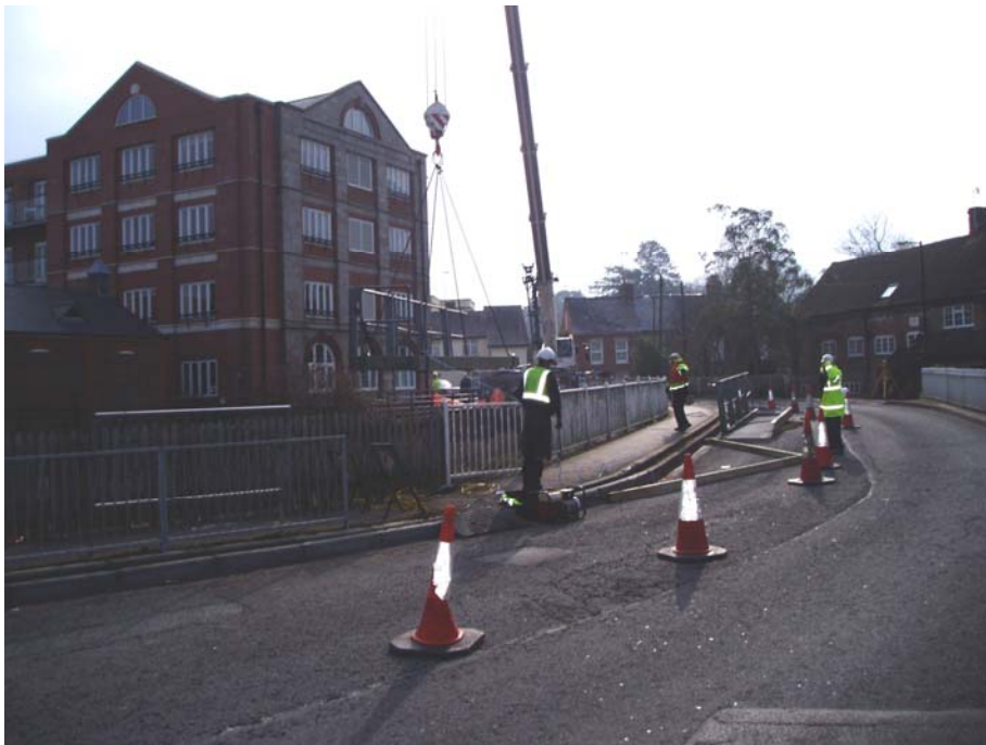
Photo 3 – Removal of Environment Agency walkway
