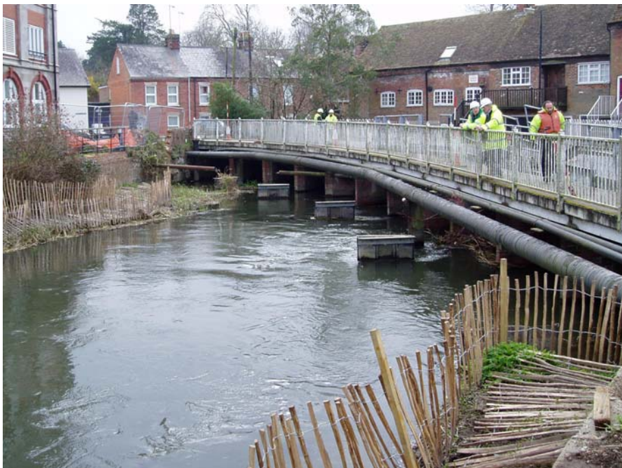
Photo 4 – Tannery Bridge following removal of Environment Agency walkway
