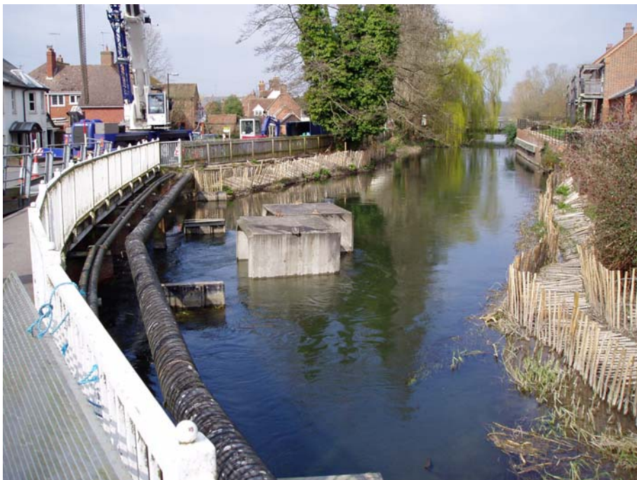
Photo 6 – Footbridge centre pier in place
