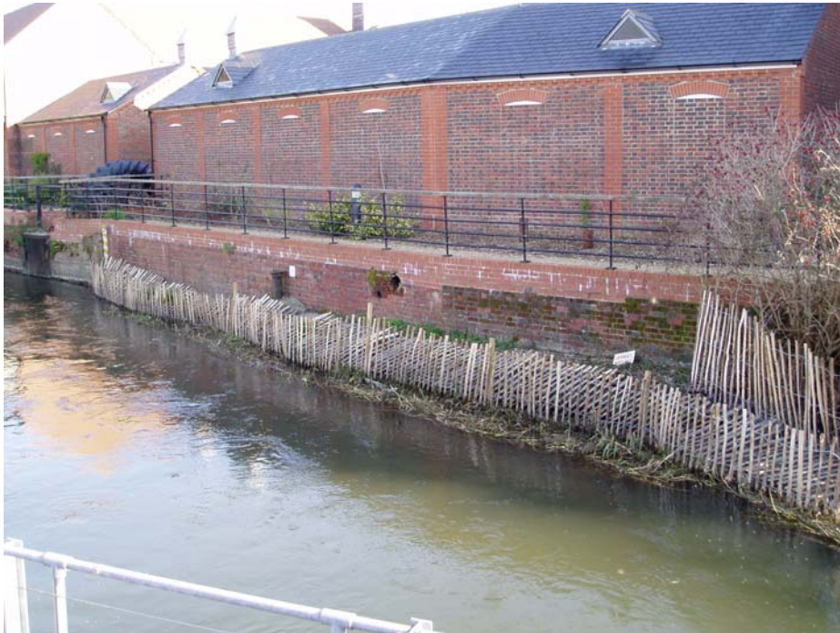
Photo 1 – Chestnut fencing installed to upstream banks
