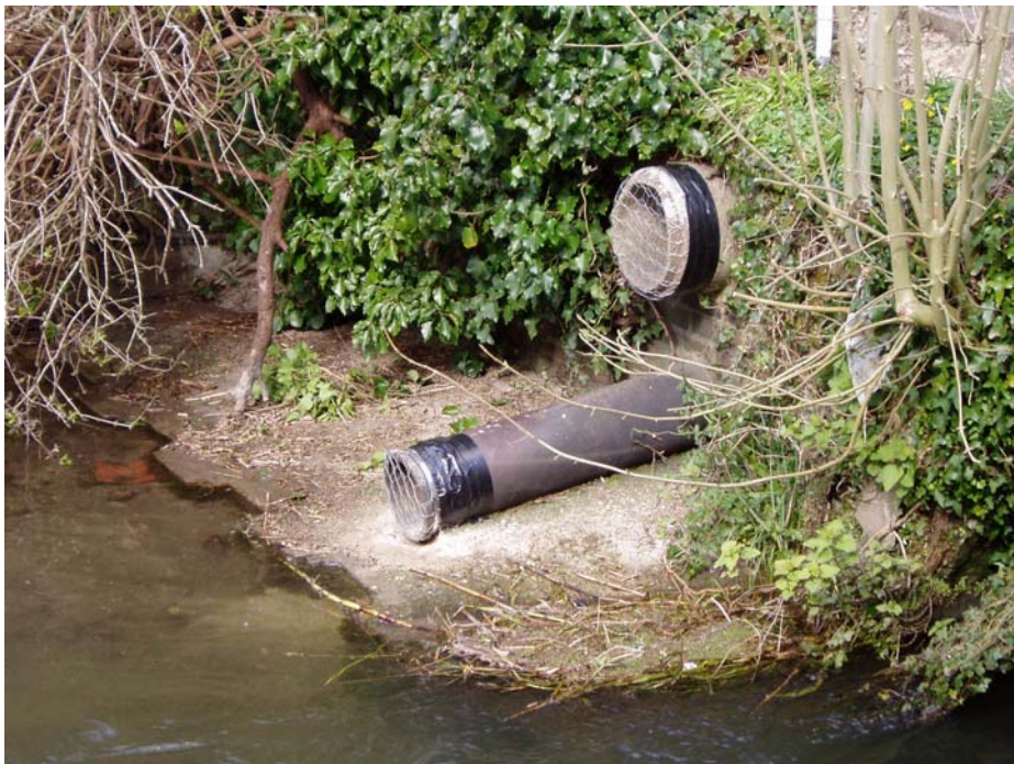
Photo 2 – Highway drainage pipes in Waterside
