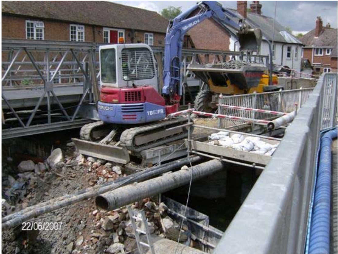
Removal of excavated material
