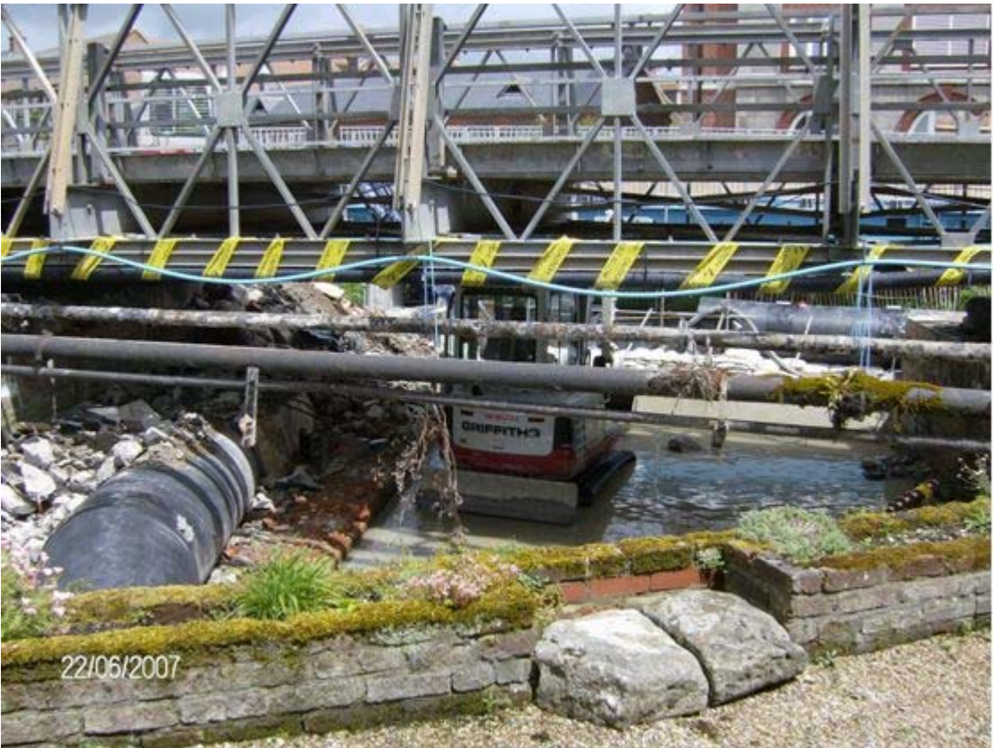
Excavation of spans 5 -7
