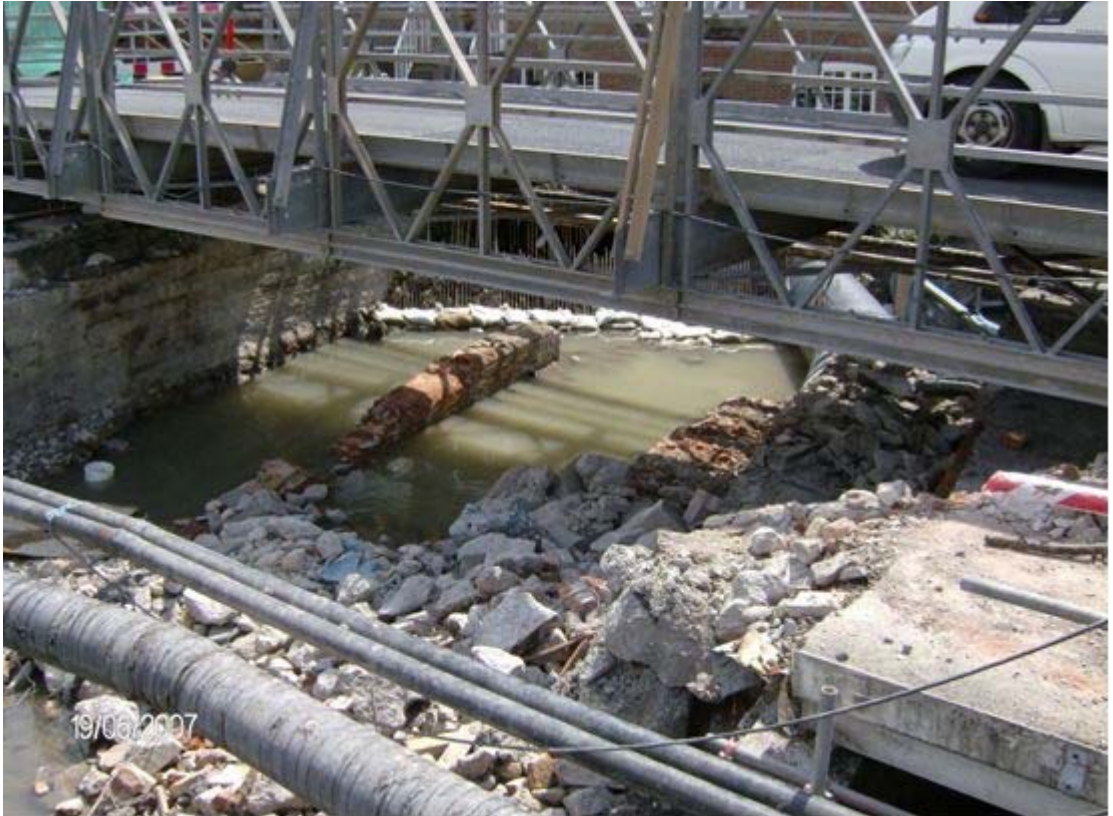
Demolished spans 5 -7: deck debris removed
