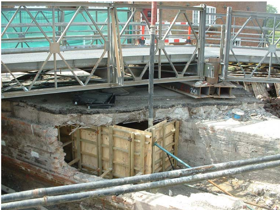
Area where concrete is being placed (underneath the temporary road bridge)
