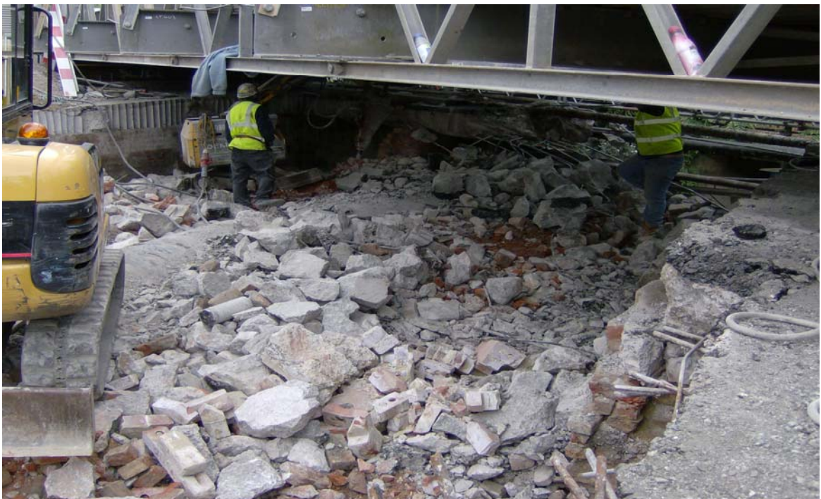
Demolition to Spans 1 – 3 Including Piers 1/2
