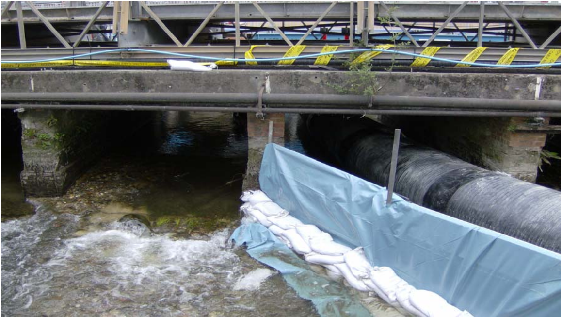
Dam Construction – Rear of Span 7
